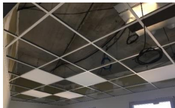
Pose des dalles Eurocoustic © Saint-Gobain Eurocoustic
